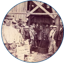
Tunnel workers ready to descend the Central Shaft
